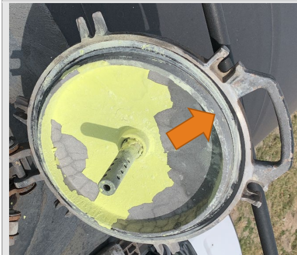
Figure 11 - Manway cover gasket
