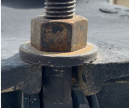
Figure 14 - Eyebolt flat washer
