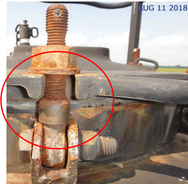
Figure 18 - Collar not engaged with lid. Do not ship
