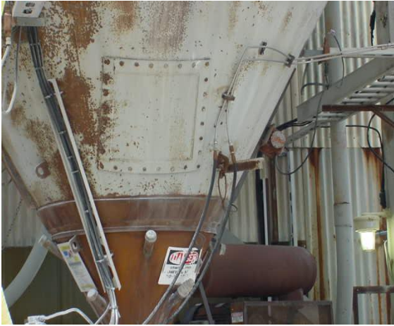
Bin – This is a confined space.
