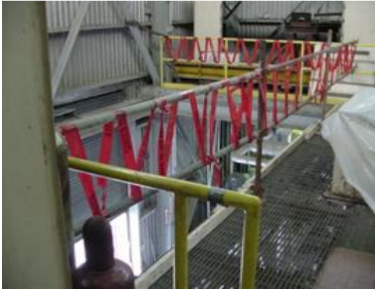
Pictures of Properly Protected Openings. Refer to the Phosphates Walking/Working Surfaces Program for detailed requirements.
