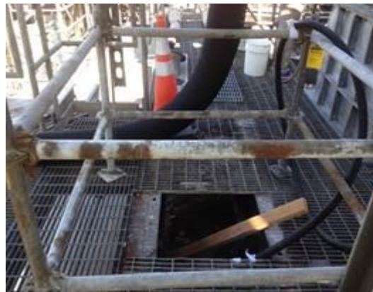
Pictures of Properly Protected Openings. Refer to the Phosphates Walking/Working Surfaces Program for detailed requirements.
