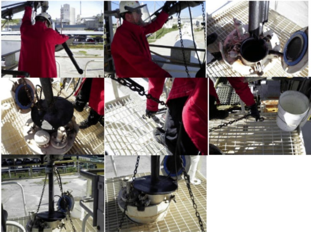
Figure 21 – Inset loading spout and secure loading arm
