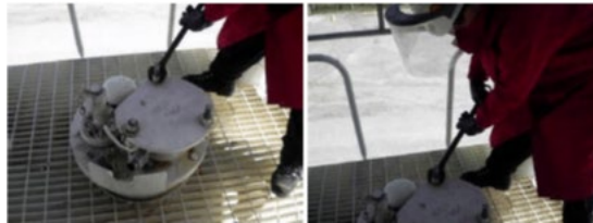
Figure 25 - Close manway and tighten bolts
