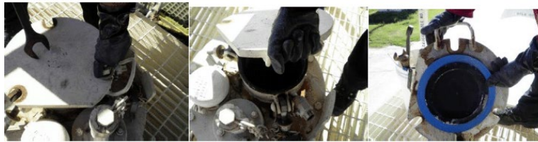
Figure 17 - Inspect manway gasket
