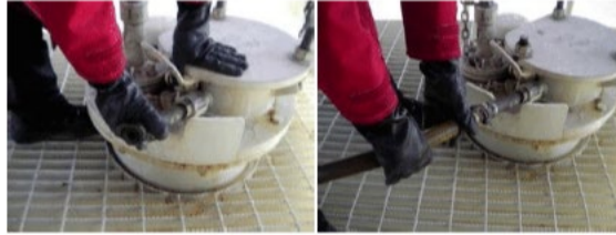
Figure 26 - Connect air supply for pressure test
