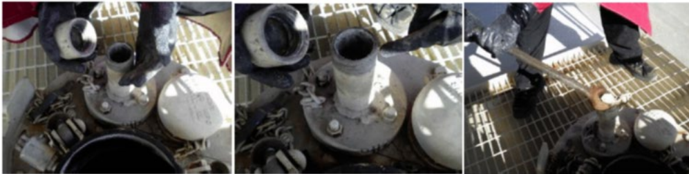
Figure 20 - Inspect Product Siphon Cap and Gasket
