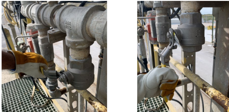
Figure 28 – Relieve air pressure before disconnecting air supply from car dome
